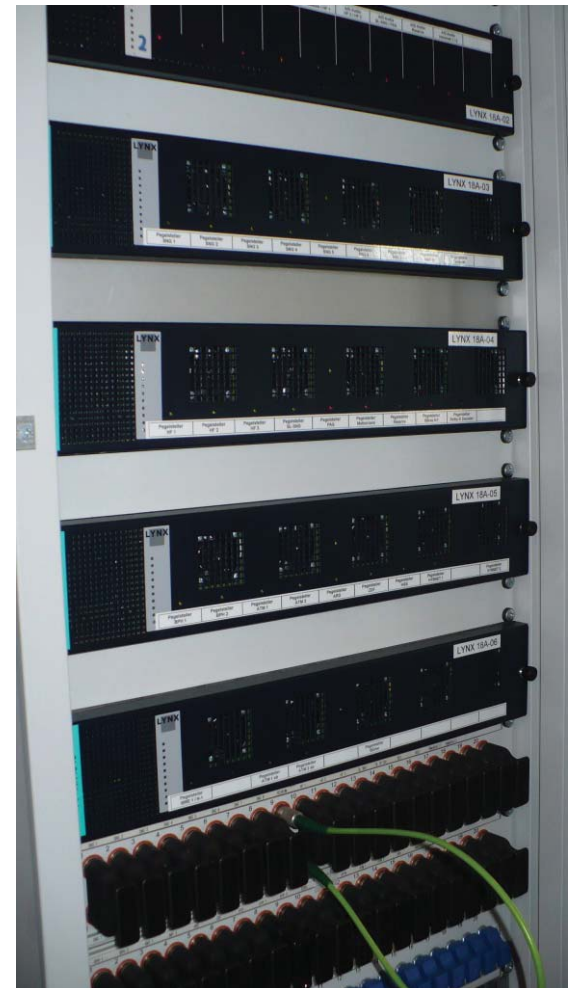
LYNX Series 5000 Racks installed at DW-TV
