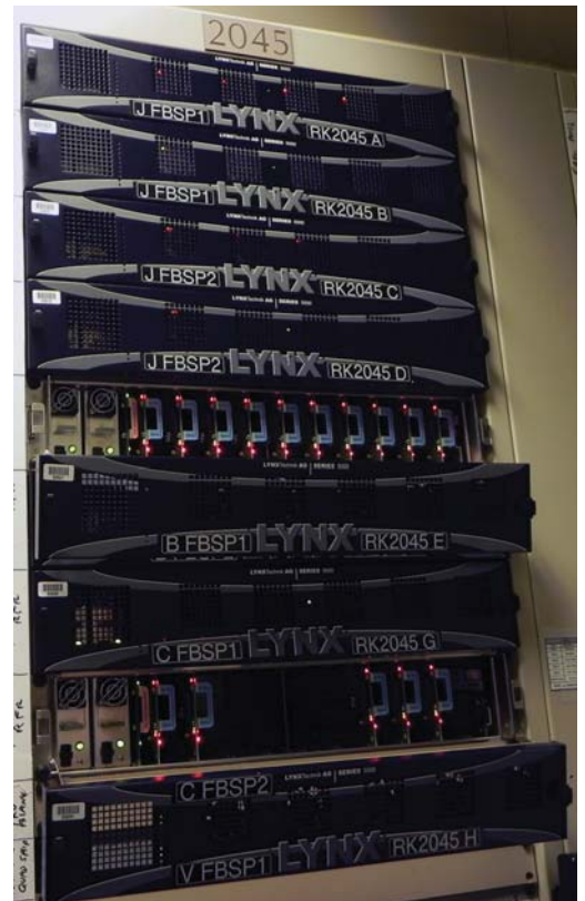
Rack of LYNX Technik Series 5000 cards
